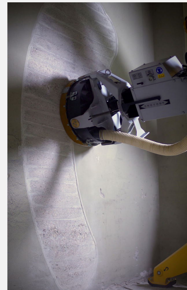
Stripping – preserves building fabric and reduces disposal costs
